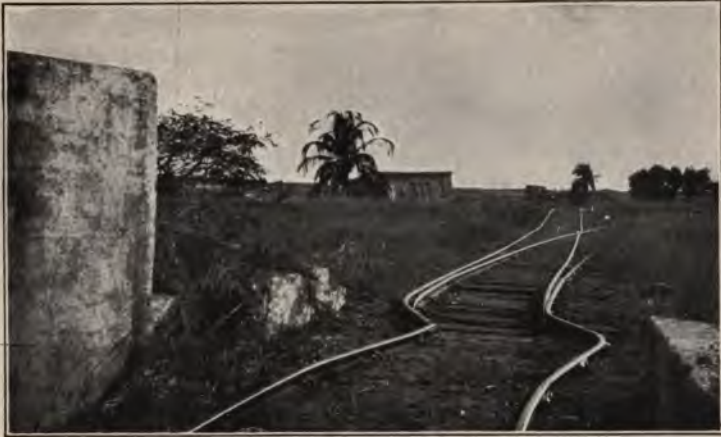
A. Subsidence of the ground with consequent tilting of buildings in the Victoria Battery, Port Royal. The kink in the railway track is over a fault.
